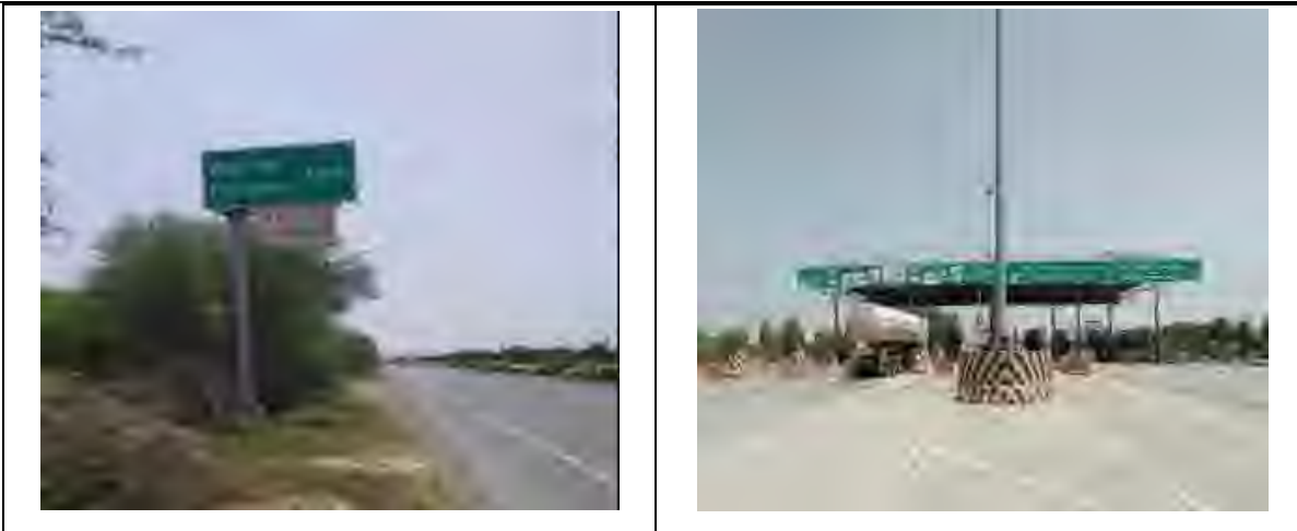
Figure 2-2 : Photographs showing Project Corridor
