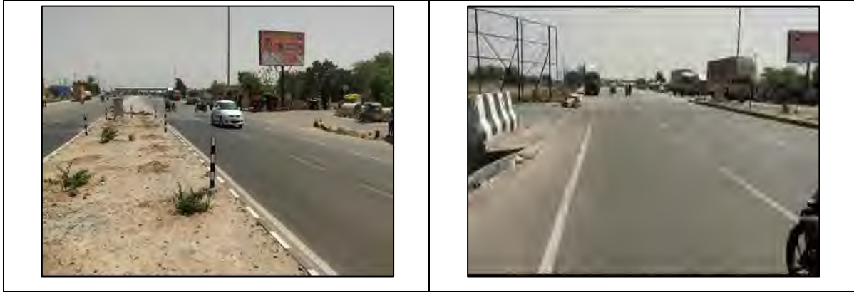
Figure 2-2: Photographs showing Project Corridor
