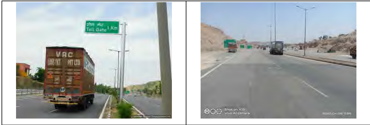
Figure 2-2 : Photographs showing Project Corridor
