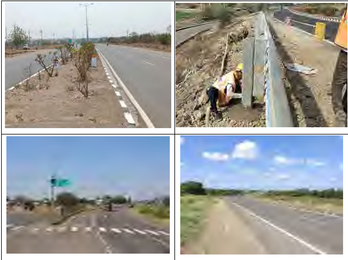
Figure 2-2: Photographs showing Project Corridor
