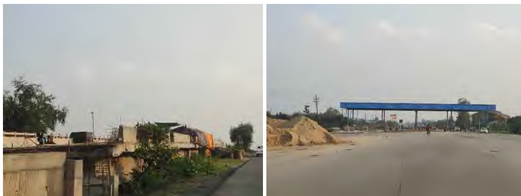
Figure 4-5 ROB & Toll Plaza under construction
