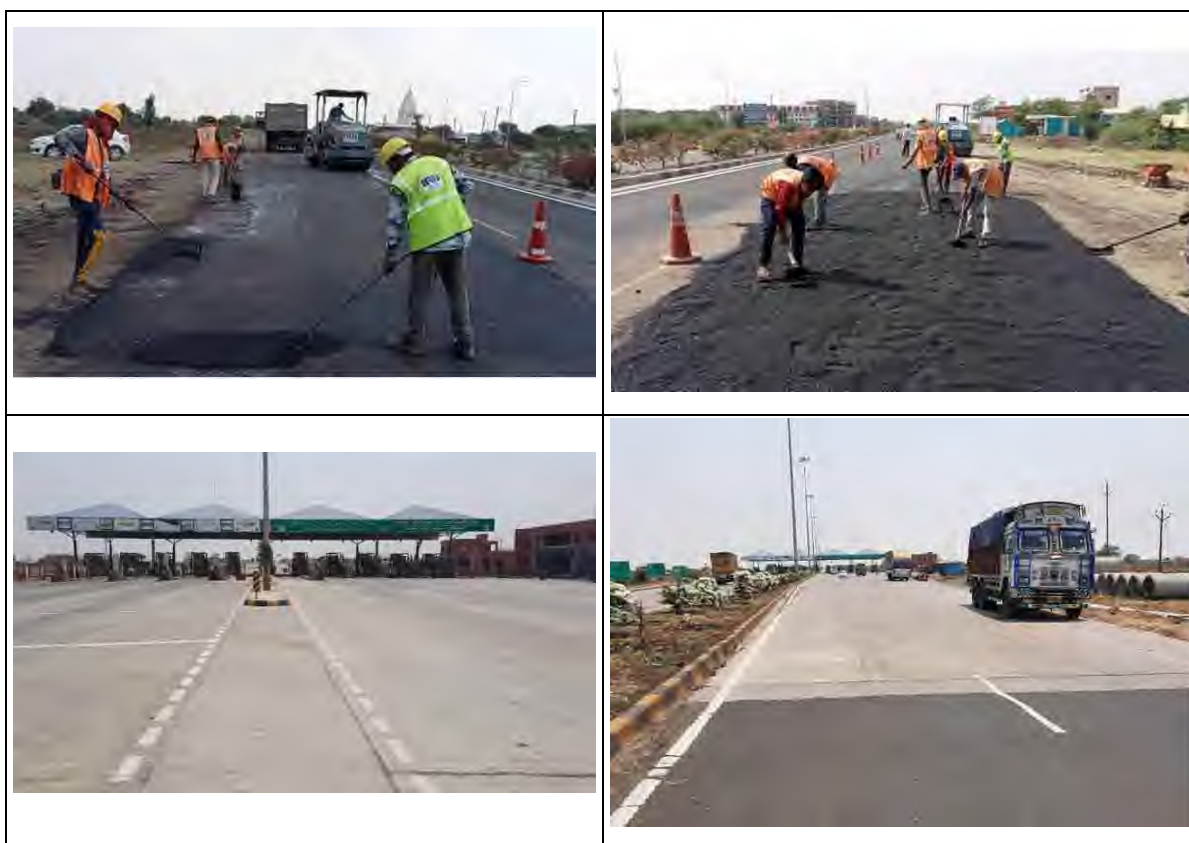
Figure 2-2 : Photographs showing Project Corridor
