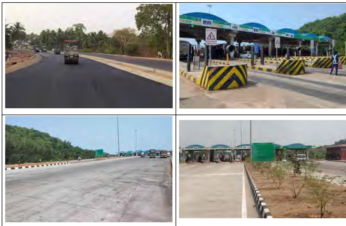
Figure 2-2 : Photographs showing Project Corridor
