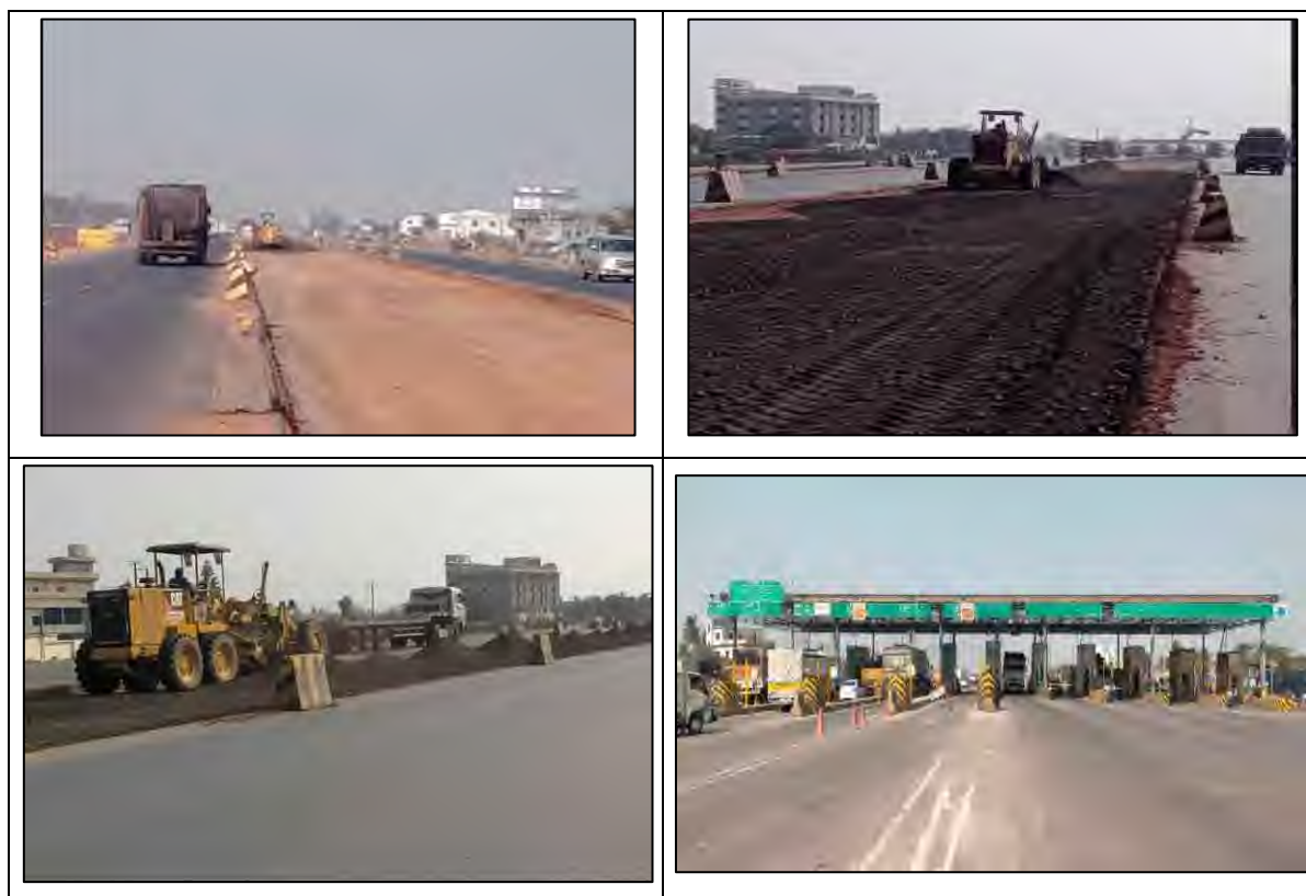
Figure 2-2: Photographs showing Project Corridor
