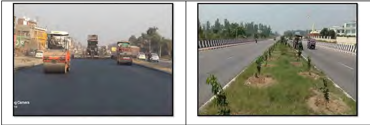
Figure 2-3: Photographs showing Project Corridor
